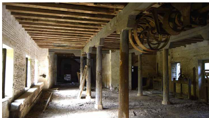
Figure 2. Ground floor with machinery.
