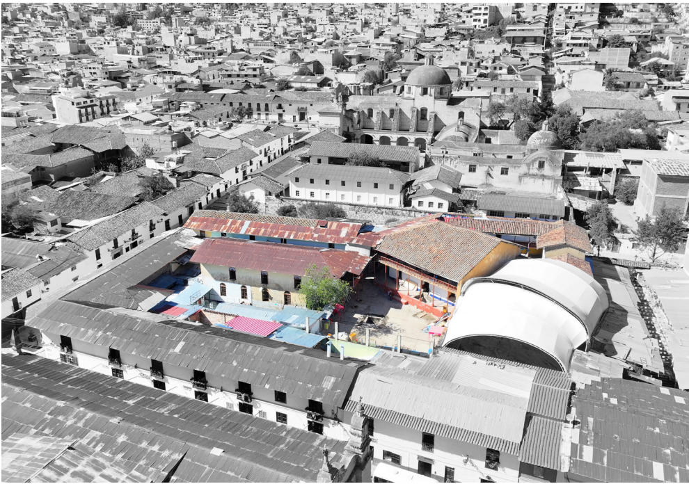
Fig. 2 Photo of the area where the land to be intervened is shown in color and the white roof covering the so-called “Cuarto de Rescate”.
