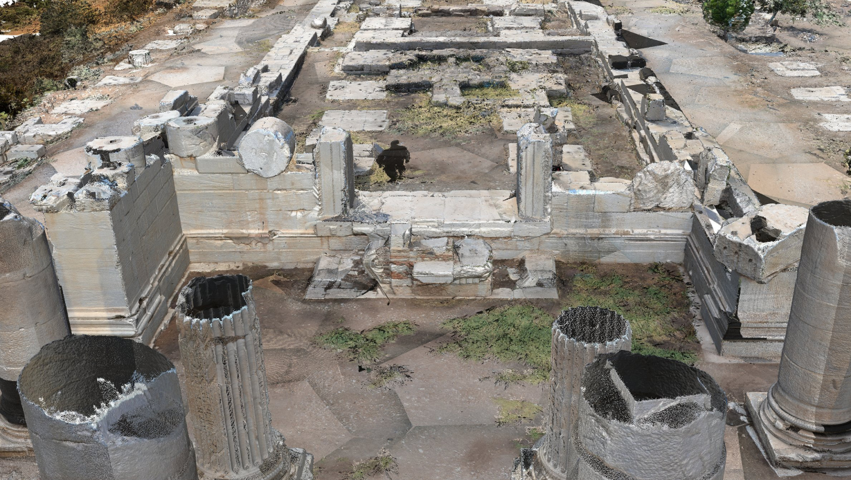
Fig. 2. Sardis, 2022 laser scans of Temple of Artemis: left, laser scan of east porch, view looking west; right, laser scan elevation of east door and wall, exaggeration of y-scale by 10 times revealing hidden curvatures in the masonry.
